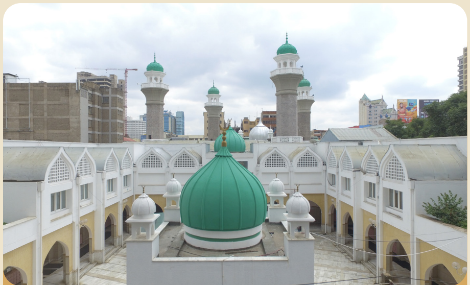
Jamia Mosque Nairobi after the extension
